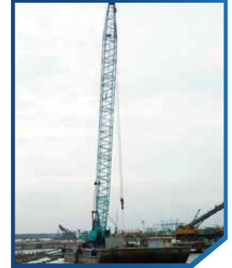
Equipment: Crawler Cranes 100 - 125T Origin: Japan (IHI, KH) Quantity: 04
