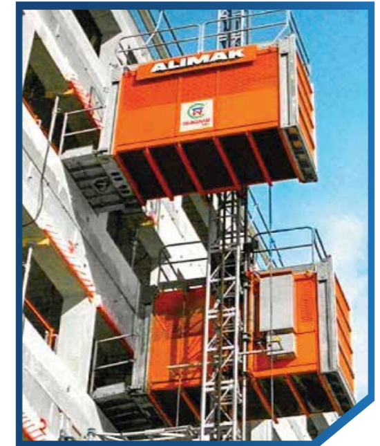
Equipment: Construction Elevator Origin: China Quantity: 03 Function: Transporting workers and materials to high elevations
