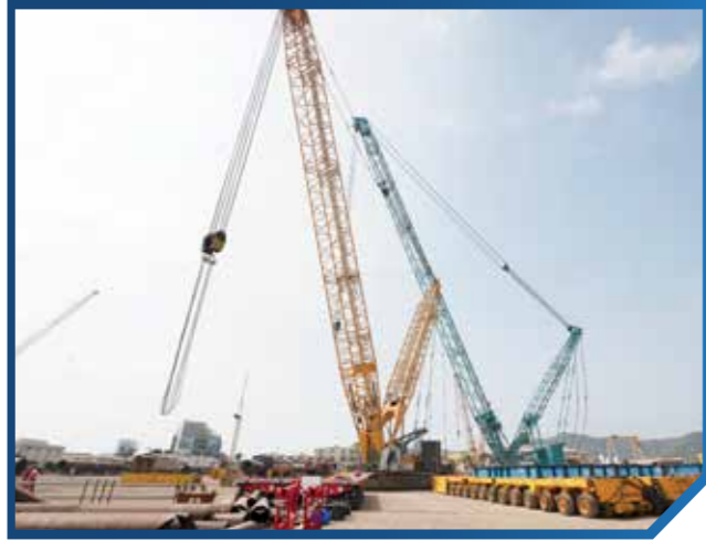
Equipment: Crawler Crane 750T Origin: Germany Quantity: 01
