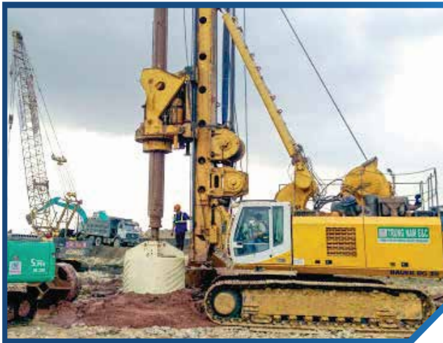
Equipment: Bauer (BG36) Bored Piling Rig Origin: Germany Quantity: 03
