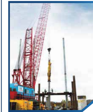
Equipment: Crawler Cranes Lima 240T Origin: Japan Quantity: 03
