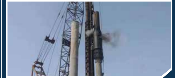
Equipment: 3.5T Diesel Hammer Origin: China Quantity: 10 Function: Driving DUL reinforced concrete D500A piles
