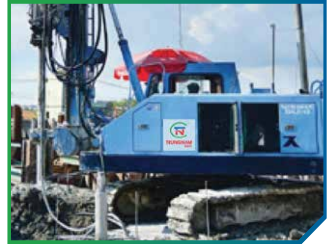
Equipment: XMD Bored Piling Rig Origin: Japan; Quantity: 04 Function: Drilling for pier and abutment foundations
