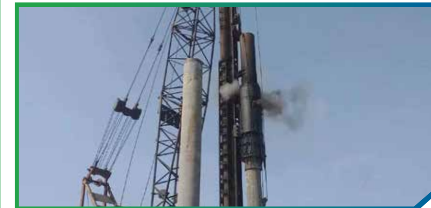
Equipment: 3.5T Diesel Hammer Origin: China Quantity: 10 Function: Driving DUL reinforced concrete D500A piles
