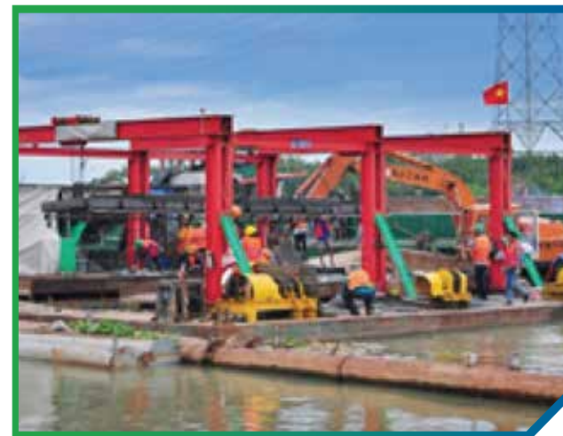
Equipment: Stone carpet machine Origin: Vietnam Quantity: 04 Function: Stone carpet to reinforce the riverbed
