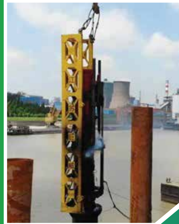
Equipment: 2.5T Diesel Hammer Origin: China Quantity: 06 Function: Driving DUL reinforced concrete D350A piles
